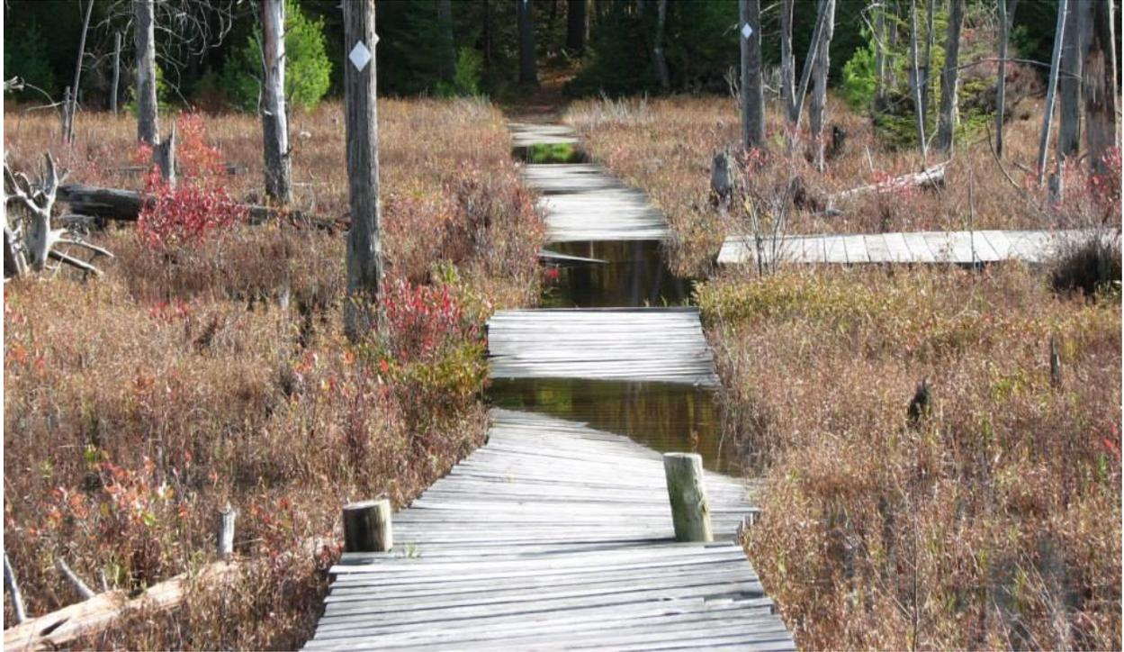
The boardwalk across Dustin Swamp, shortly after the beavers moved in. Their activities caused flooding, which in turn caused significant damage to the boardwalk.
